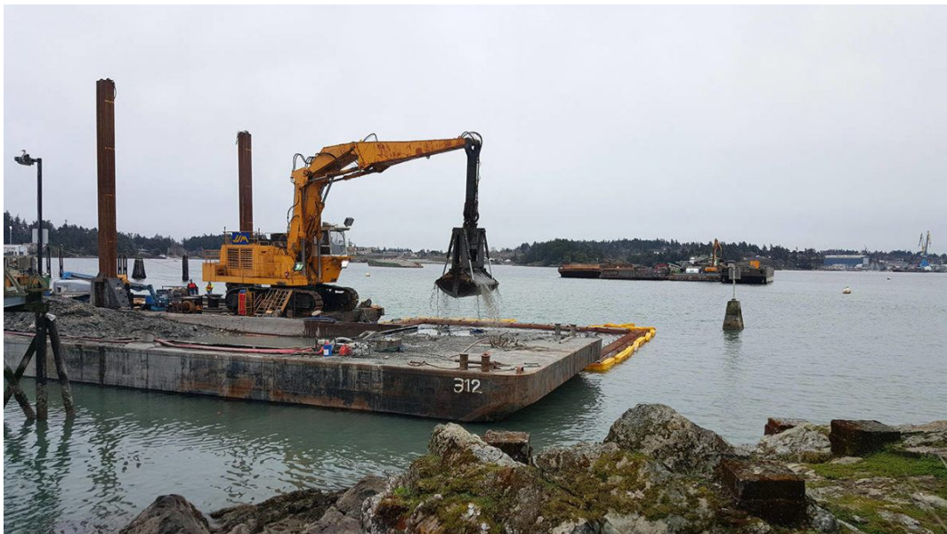
An excavator dredges sediment from the Esquimalt Harbour. Photo from Victoria News, April 7, 2017, courtesy of CFB Esquimalt.
